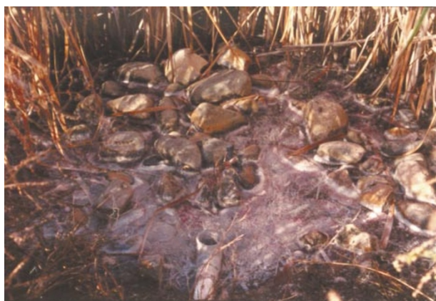
Fig. 4 Photograph of purple and white S-oxidizing bacteria near the outlet distribution pipe for cells 2 and 3. The purple bacteria are incompletely oxidizing H 2 S to elemental sulfur. Similar growths of purple bacteria have been reported for H 2 S-rich effluent waters at other constructed wetlands (James Gusek, personal communication, 1999). Although bacterial identification was not attempted in this study, it is likely 78 that the purple microbes include the Chromatiaceae and possibly Rhodospirillaceae , whereas an anonymous reviewer of this article suggested the filamentous white bacteria could be Beggiatoacea .
